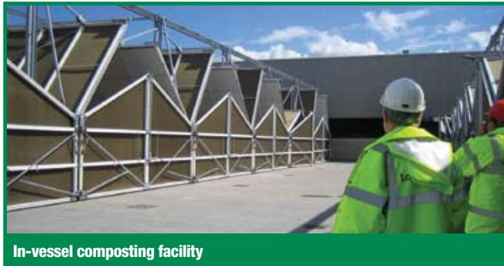
In-vessel plants are more commonly constructed in areas where other users are sensitive to potential odours as much greater control of the emissions can be achieved than is possible with windrow facilities.
